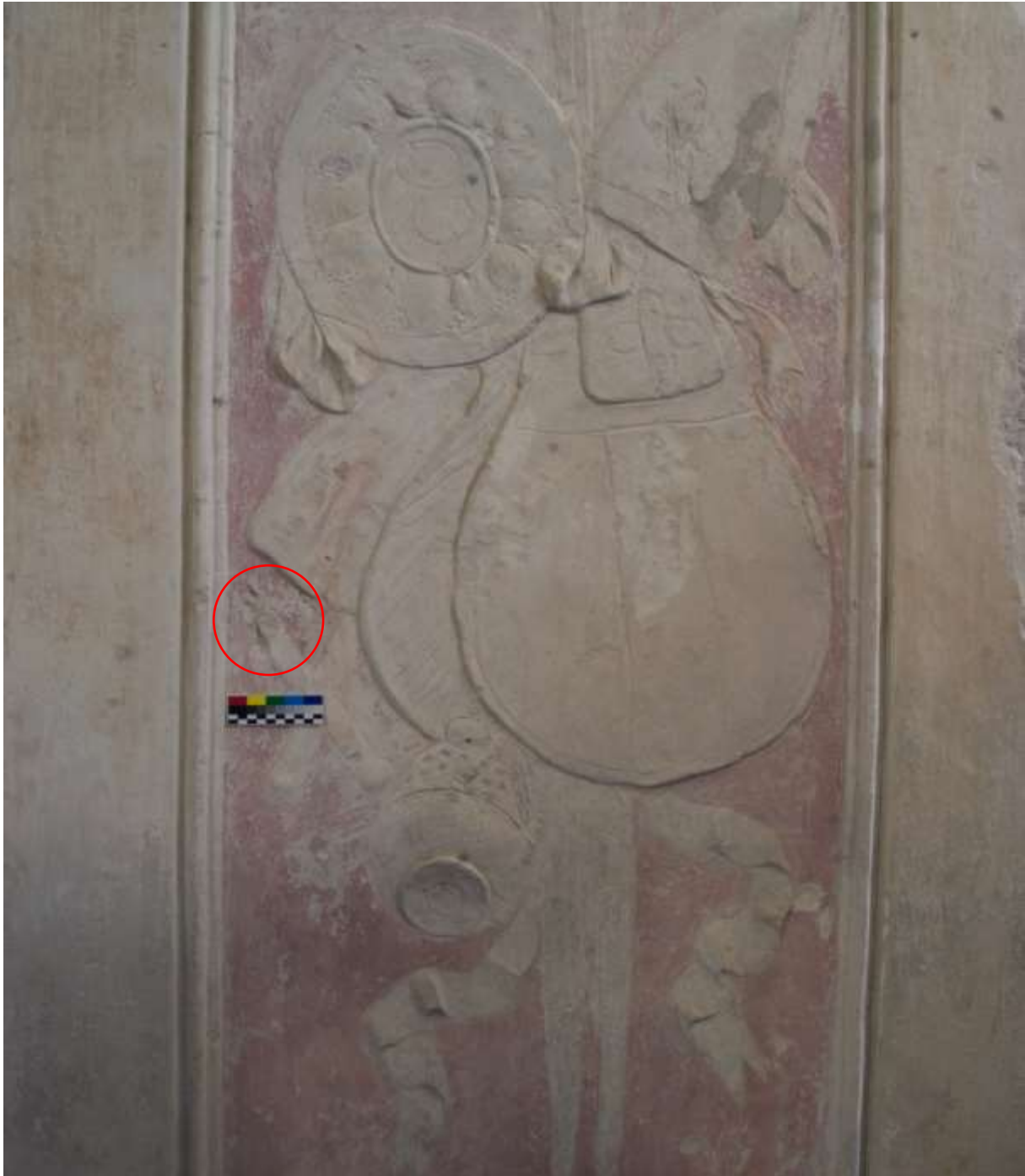
Figure 18. Transition between the plastic part and the flat background. Extraction site of sample SDOB 2.
