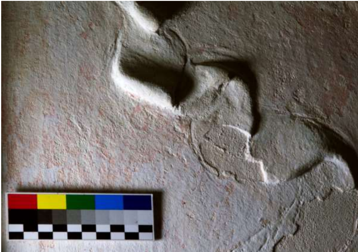
Figure 1. Plastic ribbon, sample of stucco. Extraction site of sample SDOB 1.
